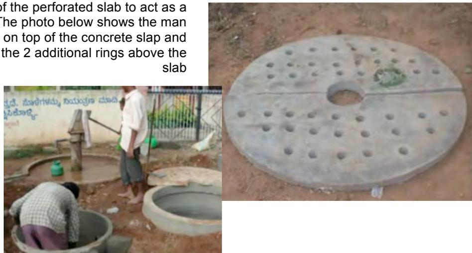
3. The 2 rings on top of the concrete slab are filled with 20 centimeters filtering medias:
