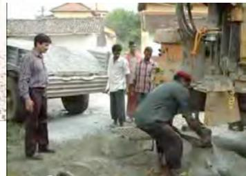
**2. Filling up of the borer well with small gravel to the height of 5 feet (1.52 meters)**
