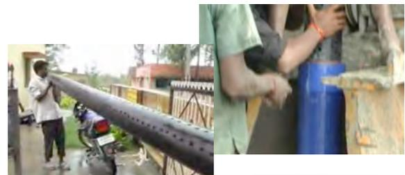
**4. Once the pipe is placed inside the borehole, gravel is placed to fill the space around the hole.** Stormwater can now be oriented to it.
