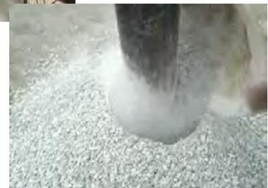
Figure 5. Example of wells either installed or refitted used for aquifer replenishment by gravity-fed wells: Here wells are 5 feet diameter (1.52 meters) and 15 feet deep (4.57 meters).
