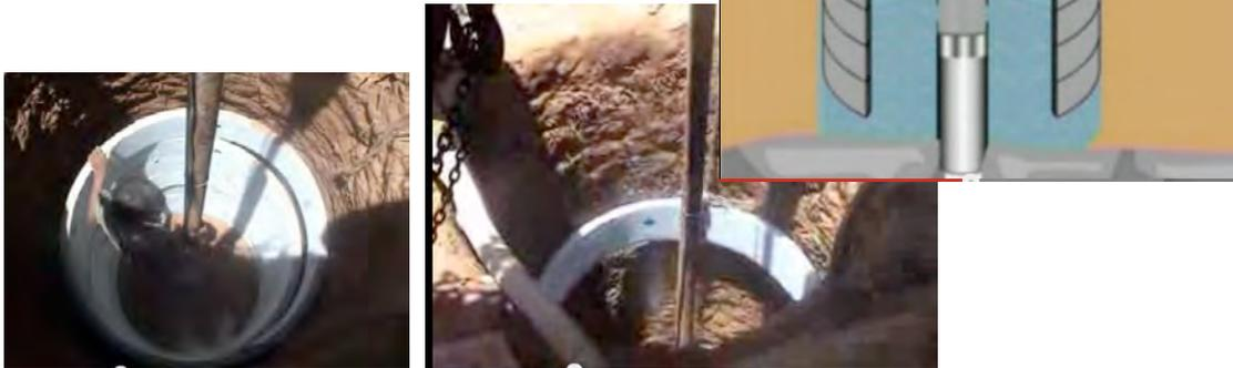
2. Once all the 13 rings have been placed, a perforated reinforced concrete slab is placed on top and then 2 more rings are placed on top of the perforated slab to act as a filter. The photo below shows the man standing on top of the concrete slab and installing the 2 additional rings above the slab
